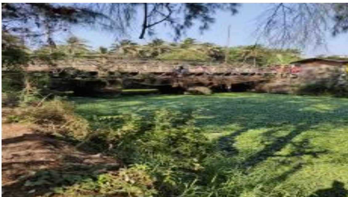
Natural outfall downstream of Khareband Bridge.
