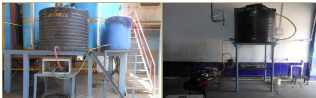
Fig No.6.10.26 & 27: High pressure pump for atomising system.
