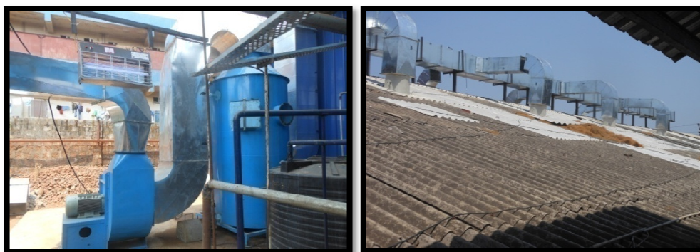
Fig No.6.10.16 & 17: Blowers and wet scrubbers arrangements
