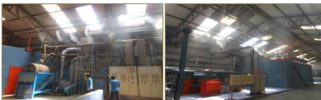
Fig No.6.10.24 & 25: High pressure atomization system
