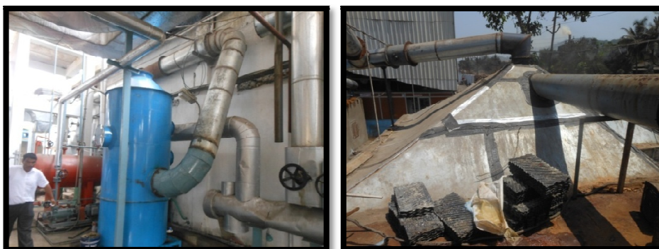
Fig No.6.10.21 & 22: Bio Filter Gas Scrubbing System
