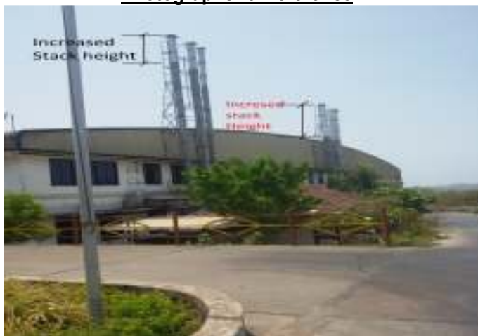
Fig6.10 (1):. Increased Stack height
