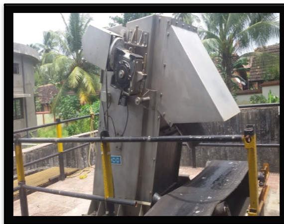
Core screen for removal of grits, plastics, metals etc. from the sewage
