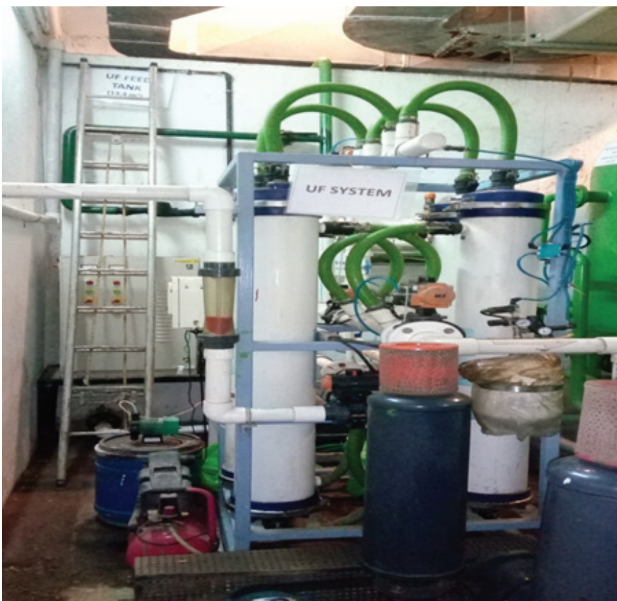
Pressure Sand Filter, Activated Carbon Filter & UV System
