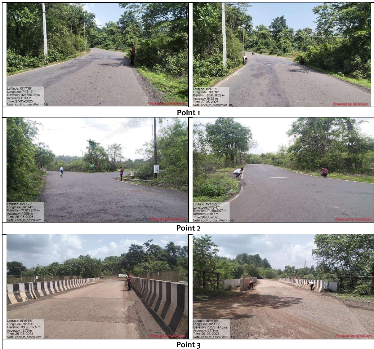
Figure 13 – Geo-tagged photographs showing Traffic Study Survey at Codli to Costi Route
